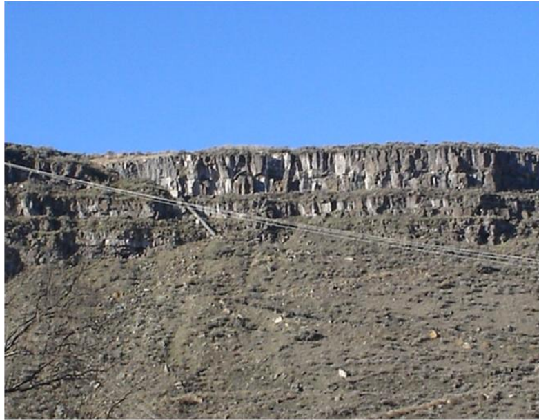
Figure 4.3.6 Twin Fall County exposed water line
